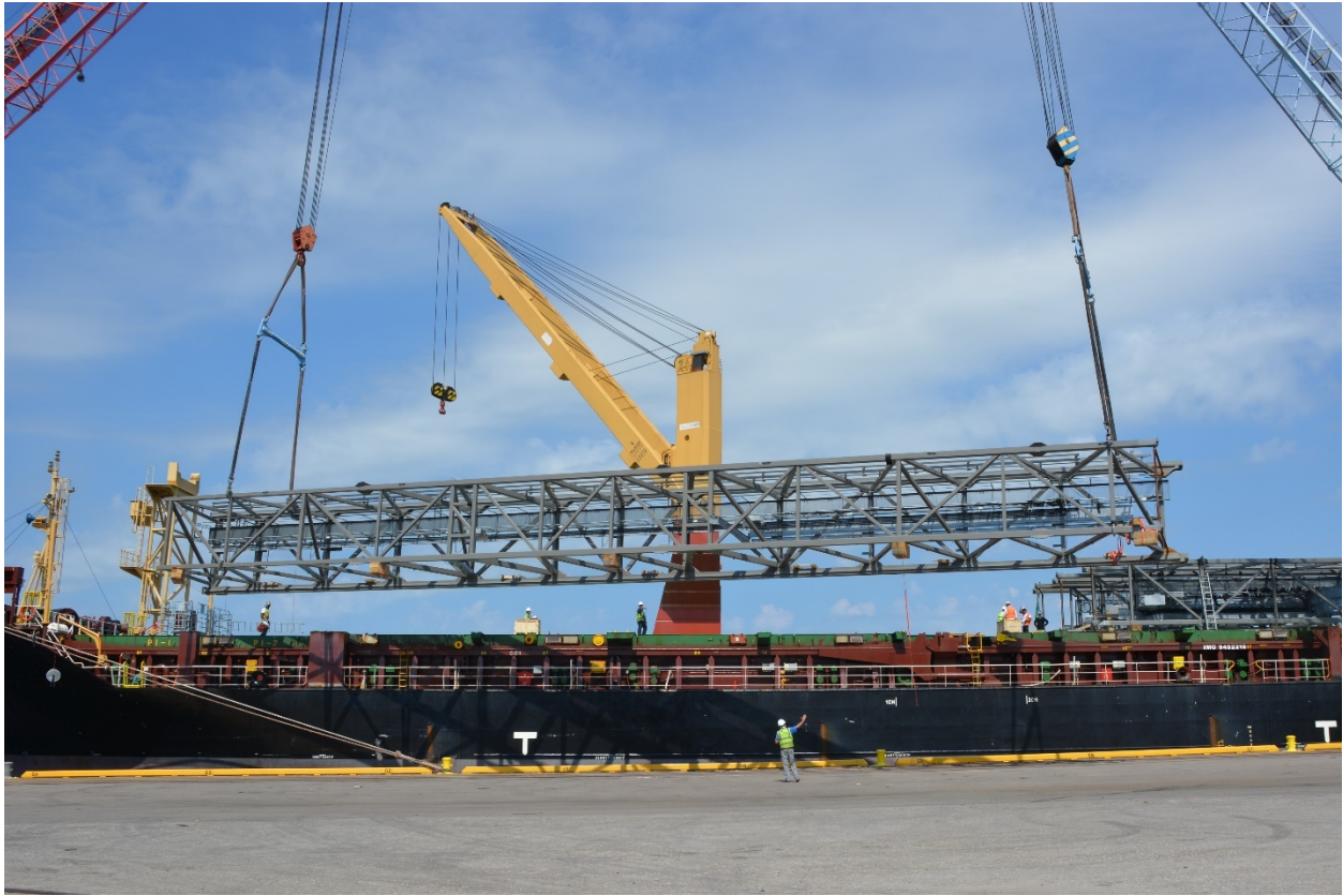
Figure 35. Crane components for CCX being unloaded at the Port of Wilmington
