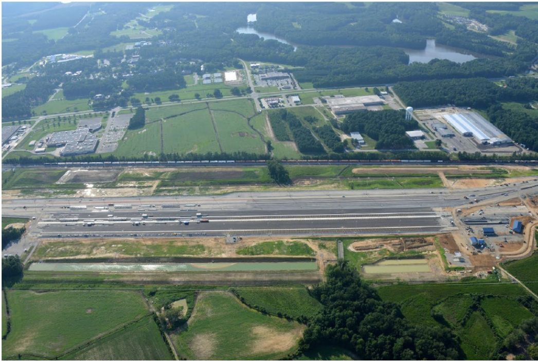
Figure 34. CCX Intermodal Terminal Under Construction (August 2020)
